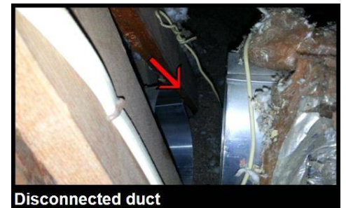
Disconnected duct
