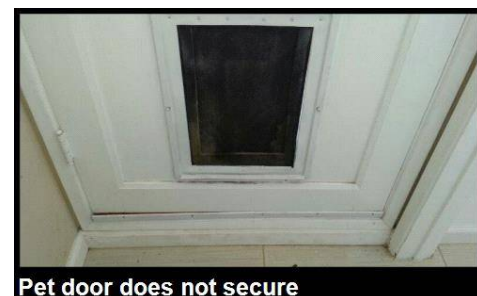
Pet door does not secure
