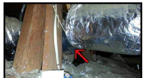
disconnected ducting
